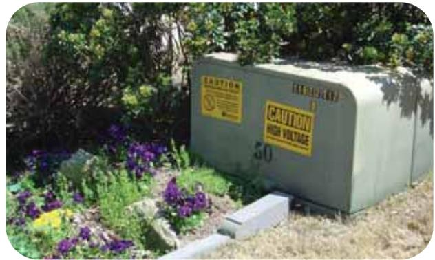
Pad-mounted transformers surrounded by vegetation or a structure may overheat and cause service interruptions when the air circulation around them is compromised. Allow at least three to four feet of space on both sides and behind the transformer.
